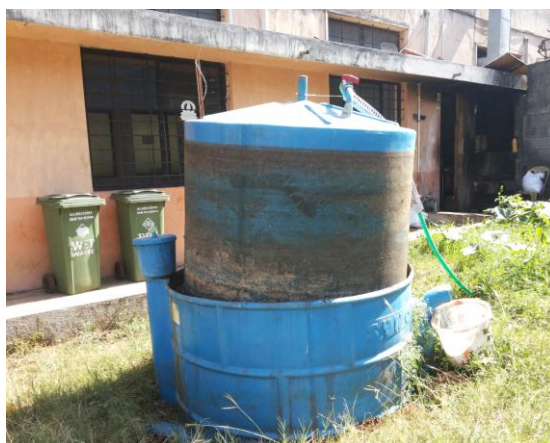
Biogas plant near canteen
